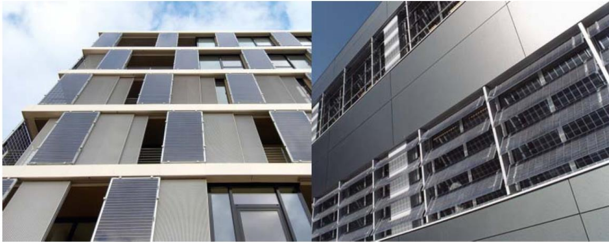
Fig. 3.B.28: solar shading solution: Left: Colt Ellisse PV sliding shades at Company HQ, Bitterfeld-Wolfen, Germany, © Colt, Right: Keuringsdienst, Eindhoven, The Netherlands, Yanovshtchinsky Architekten: using Colt Shadovoltaic as shading device, © Colt.
