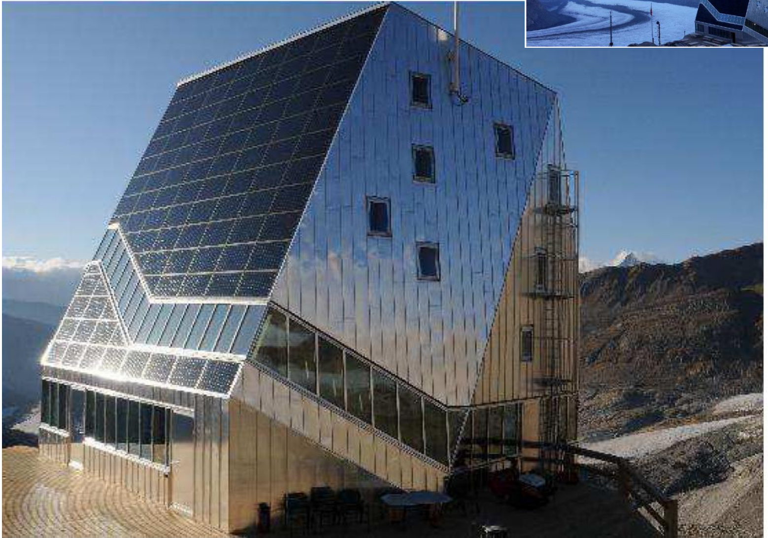
WARM FAÇADE BIPV SOLUTION, MONTE ROSA HUT (ZERMATT, SWITZERLAND) (ARCHITECT: ETH STUDIO MONTE ROSA )
