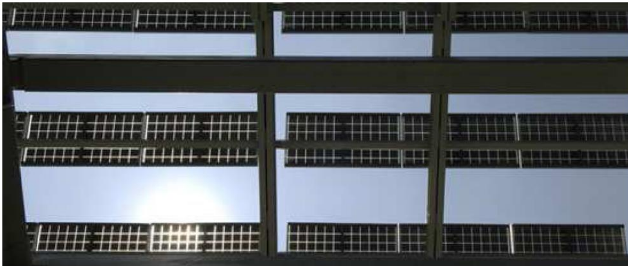
PV SHADINGS IN THE SIEEB BUILDING, BEIJING, MARIO CUCINELLA ARCHITECTS (SOURCE: WWW.SINOITAENVIRONMENT.ORG/ )
