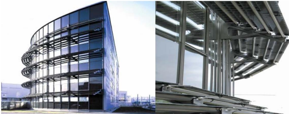
Fig. 3.B.29 SBL Offices Linz, Austria, Helmut Schimek, shading louvres with integrated photovoltaics and suntracking system, © Colt
