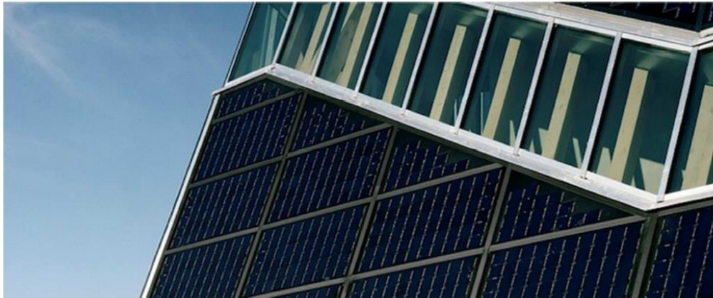
WARM FAÇADE BIPV SOLUTION, MONTE ROSA HUT (ZERMATT, SWITZERLAND) (ARCHITECT: ETH STUDIO MONTE ROSA)
