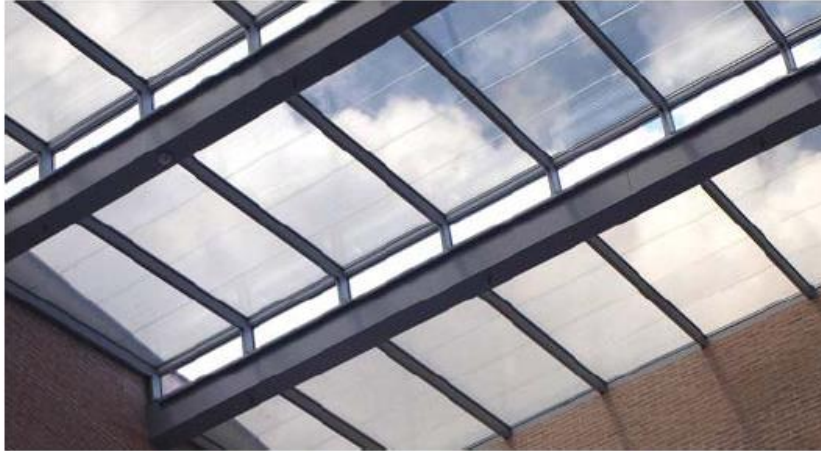
Onyx Solar Photovoltaics Transparent Glass installed into San Anton Market, Madrid (Spain)
